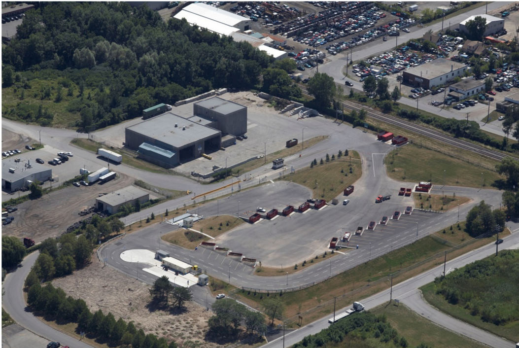
Plate 1: Typical Waste Transfer Facility
